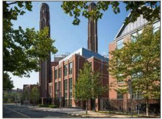
Yale Power Plant – treated in the course
